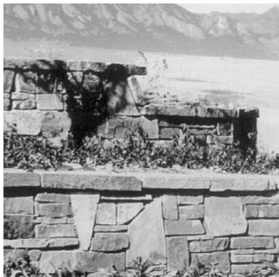
Figure 6-3 Retaining Wall Examples
