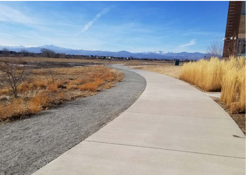
Combination Paved / Non-Paved Multi-Use Trail (12'-15')
