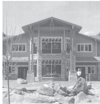
Fig. 5 - Distinguish building entrances. Notice how the pitched gable ends, supported by stone piers and posts, "announces" entrance into the senior housing building.
