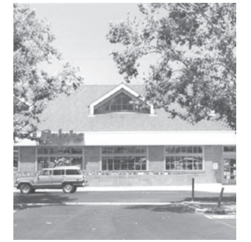
Fig. 3 - Create building transparency for all tenants. Notice how the glazed roof dormers and storefront façade optimizes interior daylighting.
