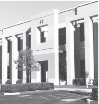
Fig. 4 - Layer wall planes. Notice how the colonnade adds layering to the façade, creating rich shadow patterns which express depth.
