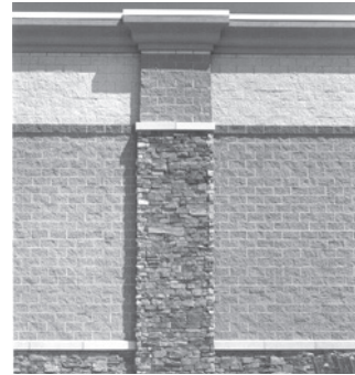
Fig. 9 - Terminate the top of Large Format buildings with a roof cap, such as a substantial cornice element that provides a building terminus while creating rich shadow lines. Notice also the ample stone pier and building base.
