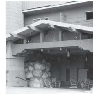
Fig. 1 - Distinguish hotel building entrances. Notice how the richly detailed pitched gable end, composed of beams and brackets, “announces” entrance into the hotel.
