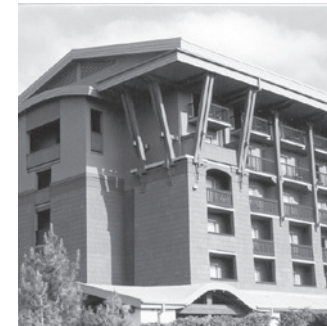
Fig. 2 - Crown hotel buildings with a discernible cap designed to terminate the top of the building. Notice how the widely overhanging eave is supported by ample brackets.
