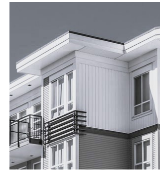
Fig. 3 - Crown office buildings with a distinctive roof cap. Notice the widely overhanging eave which terminates the top of the building.
