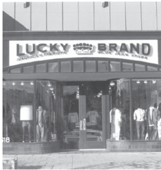
Fig. 10 - Rest Lifestyle Center buildings on a ground floor storefront composed of display windows, transoms, recessed entrances, and sign bands.
