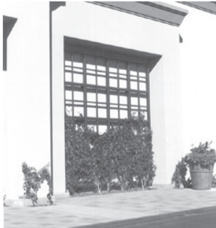
Fig. 9 - Use building recesses to add visual interest to façades. Notice how the distinctive, deeply set building recess, coupled with a trellis element, creates rich shadow patterns, enhancing façade variety.
