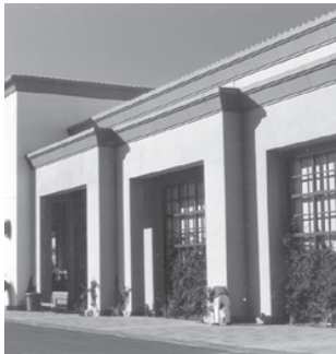
Fig. 12 - Create a distinctive cap, designed to terminate the top of the building. Notice how the distinct protruding cornice element creates a distinguishable building cap.
