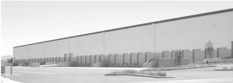
Fig. 1 - Overhead Doors and Loading Docks
