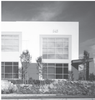
Fig. 11 - Segment building facades into a series of individual structural bays composed of piers; spandrels, and window openings.
