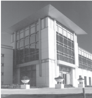
Fig. 7 - Distinguish the building entry. Notice how the entrance tower pavilion punctuates the roofscape, functioning as an identity icon while clearly identifying the building entry.
