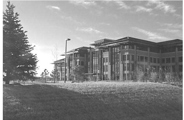
Figure 8-32 - Facades on Buildings of 4 stories or more can be broken by a combination of massing breaks and/or material changes. Note the massing breaks which create the illusion of a stepped back appearance
