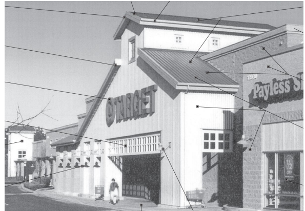
Figure 8-26 - Example of an architectural style (Target) that is more appropriate without a base. Example of integrated metal panels
