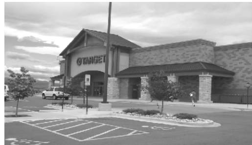
Figure 8-30 – Sloping roof forms may be used to satisfy the requirements for both “Building entrances” and “top treatments”
