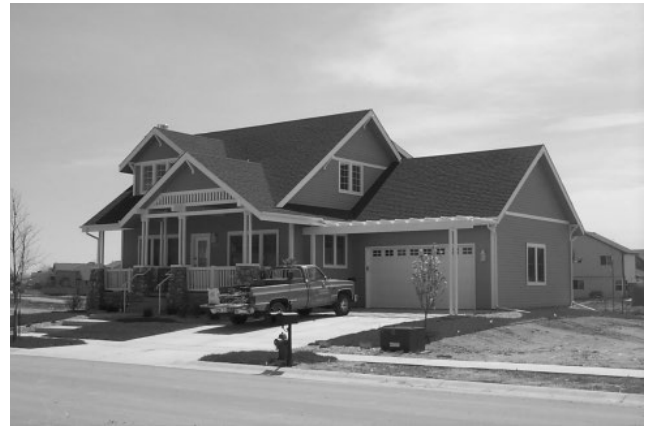
Figure 10-3 - Garage Recessed Behind the Front Façade
