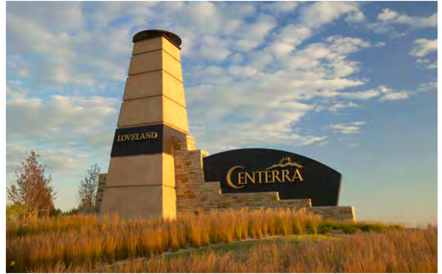
Centerra Boundary Monument
