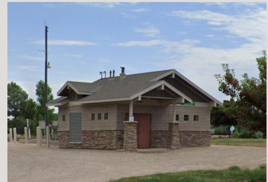
Interchange Sanitary Sewer Lift Station
