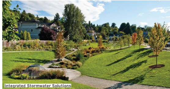
Integrated Stormwater Solutions
