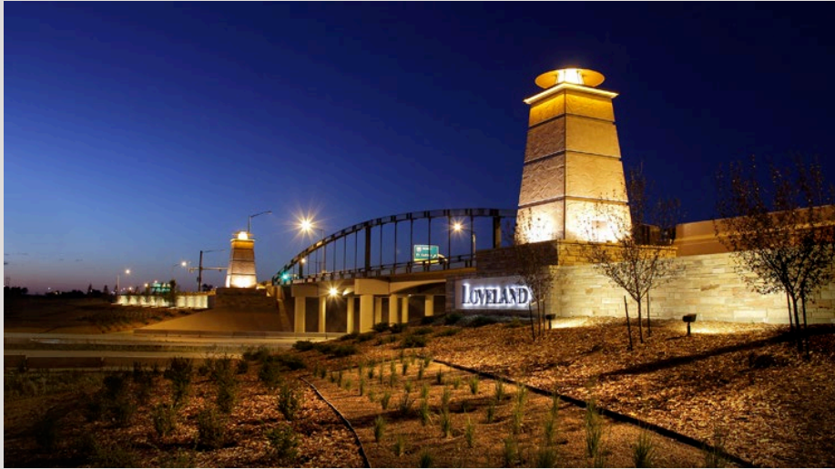
Hwy 34/I-25 Interchange (Monuments will be replaced)
