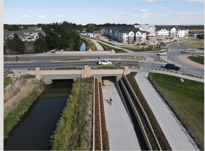
Boyd Lake Ave. and Pedestrian Underpass
