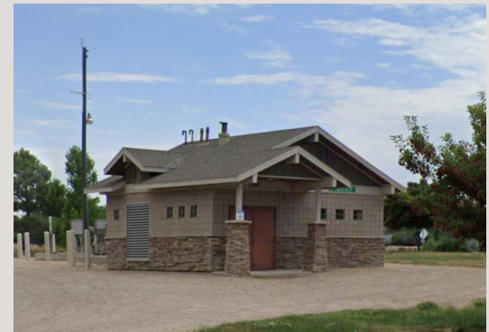
Interchange Sanitary Sewer Lift Station
