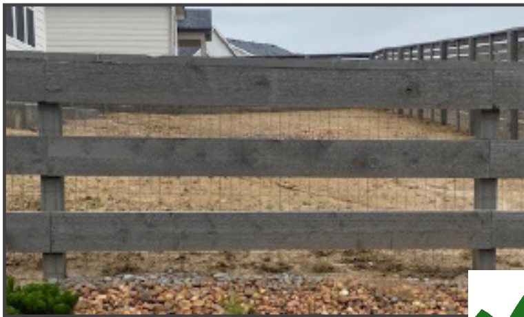
Figure 2.10O: Optional Fence Mesh (for smaller animals/critters)
