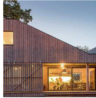
Fig. 2 - The design features a mix of modern shed and gable roof forms to create dynamic silhouettes, blending sharp geometry with clean, minimalist lines.
