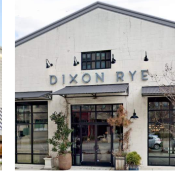
Fig. 2 - The shed and gable roof pairs with functional awnings and a calming neutral palette, creating a balanced, contemporary aesthetic.
