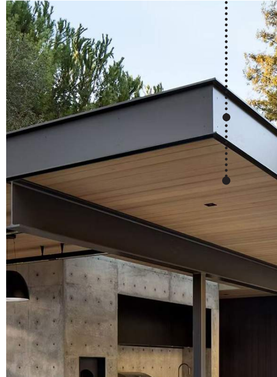
ROOFTOP STEEL CANOPY WITH WARM LINEAR WOOD UNDERSIDE HIGHLIGHTS ENTRIES, PROVIDES SHADES, AND ADDS ARCHITECTURAL INTEREST
