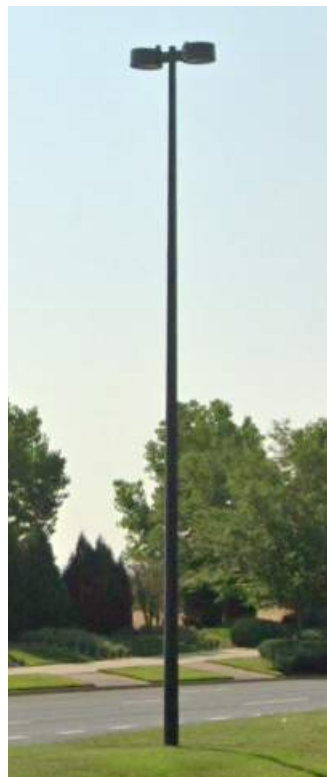
CENTERRA MAJOR ARTERIAL / MAJOR COLLECTOR STANDARD PROVIDE ROUND "HOCKEY PUCK" LUMINAIRES TO STREET LIGHTS (KIM LIGHTING CC/CSS SERIES)
