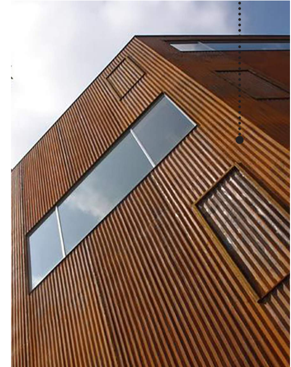
CORTEN RIBBED METAL CLADDING CREATES RHYTHM, SHADOW, AND DEPTH WHILE RELATING TO SURROUNDING MATERIALITY
