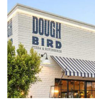
Fig. 1 - Awnings and graphics enhance the design with functional shade and striking visual elements, while lighting highlights building entry and key features.
