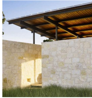
Fig. 1 - Buildings are oriented and designed to extend outward, framing an open space that aligns with the prominent market entry.
