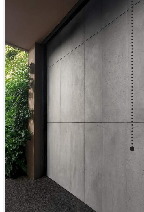
POURED-IN-PLACE CONCRETE PROVIDES HONEST, SIMPLE MATERIALITY AT ALL LEVELS
